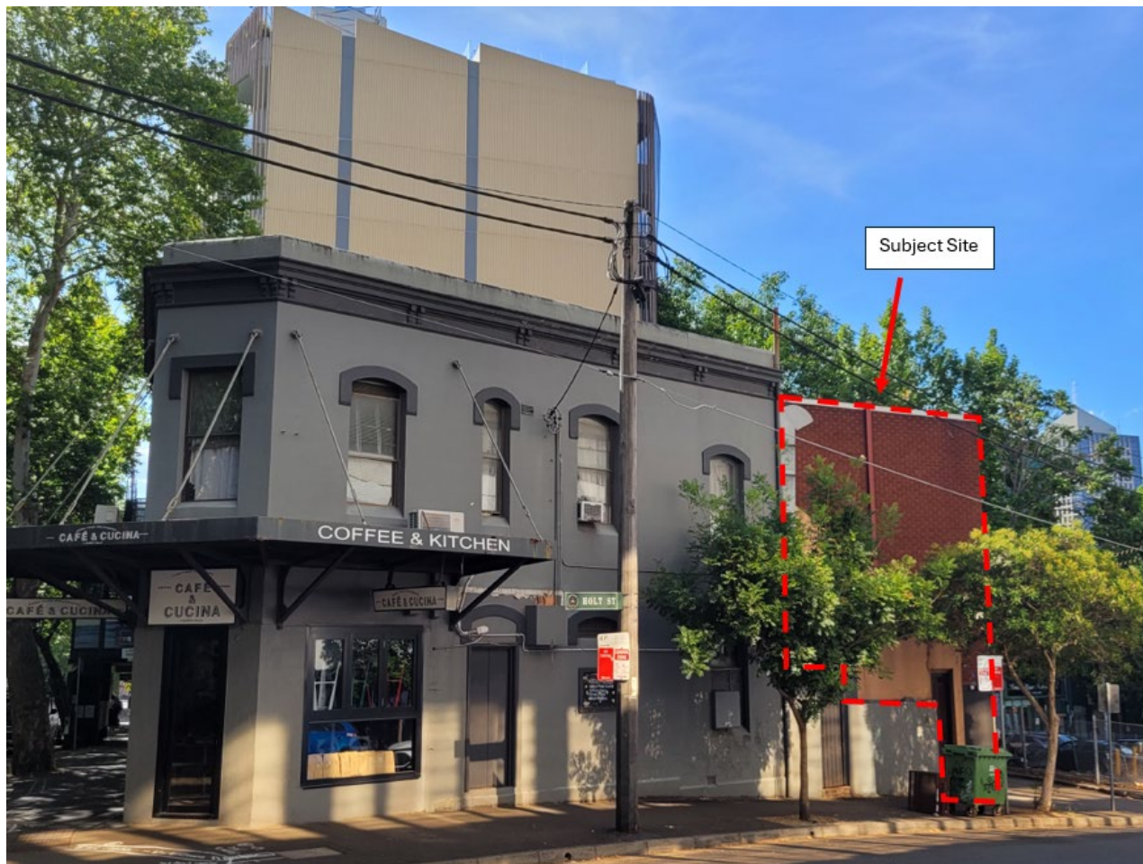
site viewed from Holt Street looking west
